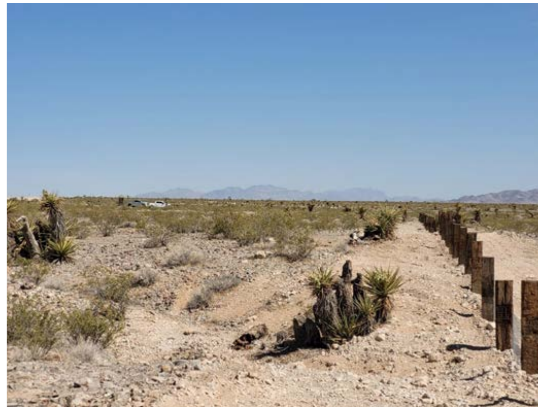
Fence alignment near Corn Creek Road.
